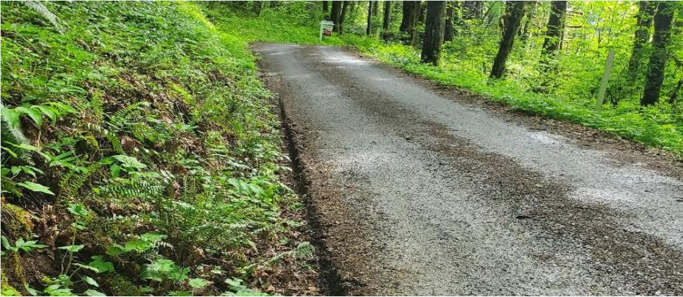
Whitman Way Culvert Cleaning
