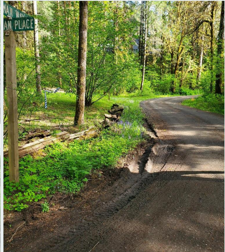
Whitman Way/Place Re-establish Ditchline 21
