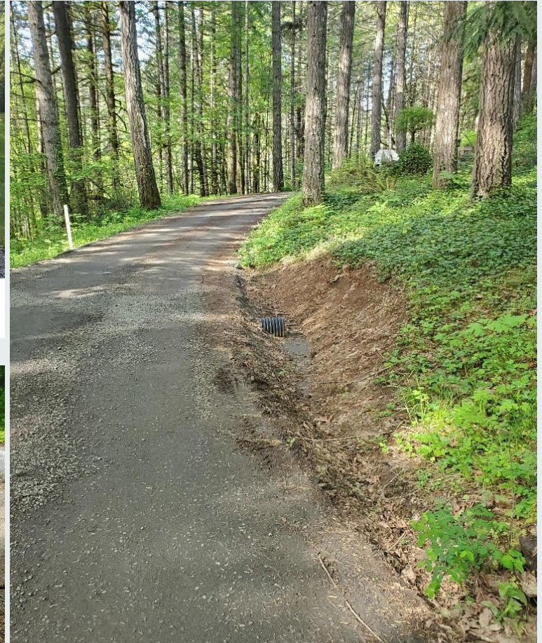
McLoughlin Culvert Install
