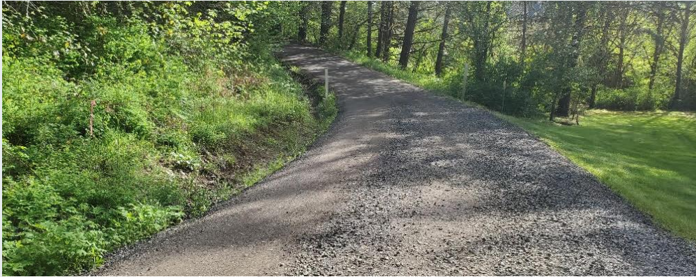
Whitman Way Rocking and Grading
