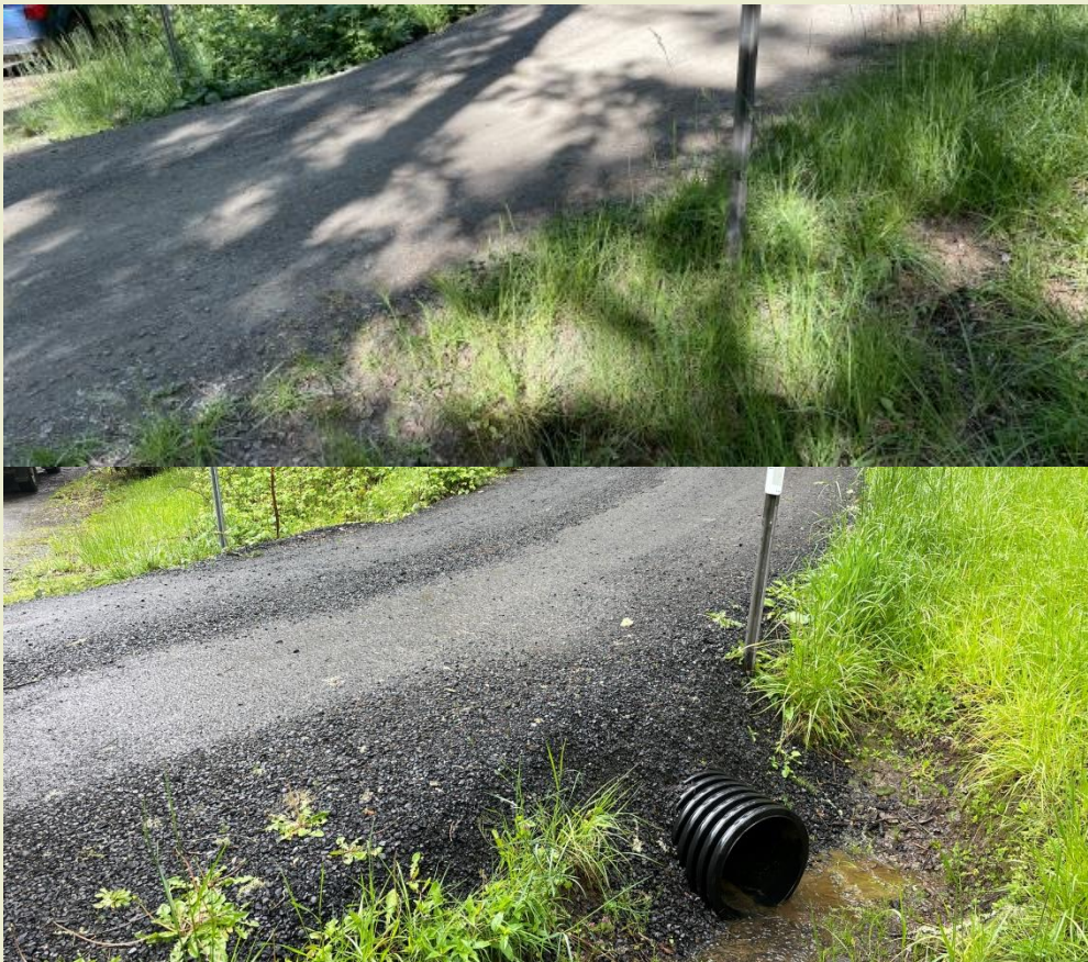
McLoughlin Drive & Whitman Way Culvert Replacements
