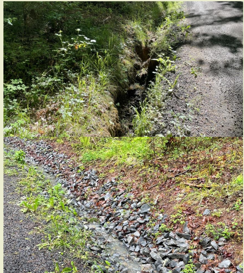
Whitman Way Ditch Repair
