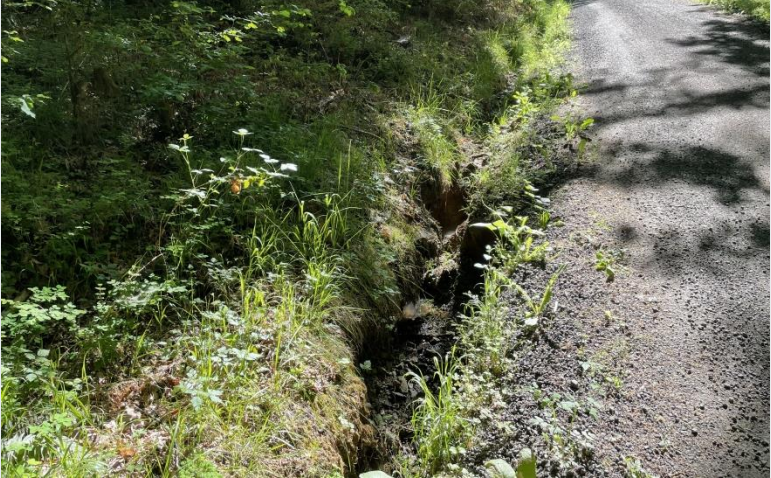
Whitman Way Ditch Repair
