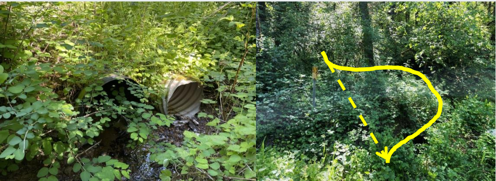
Whitman Way Culvert Inlet Repair
