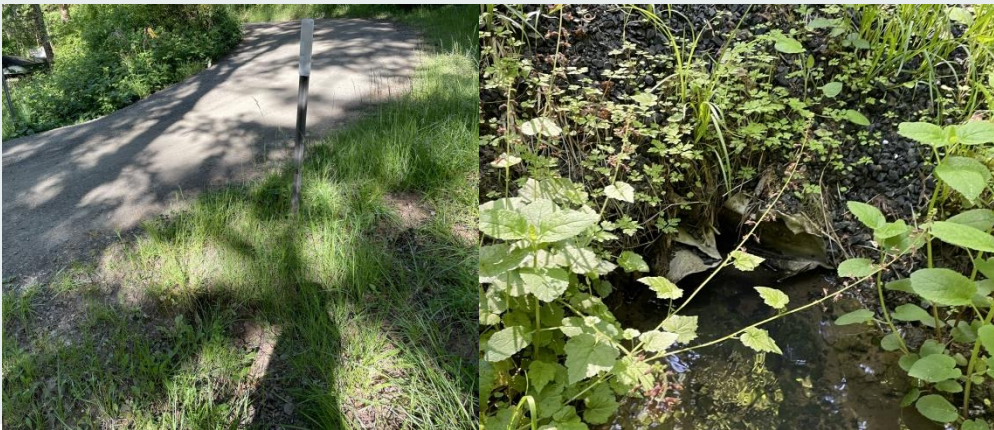
McLoughlin Drive & Whitman Way Culvert Replacements
